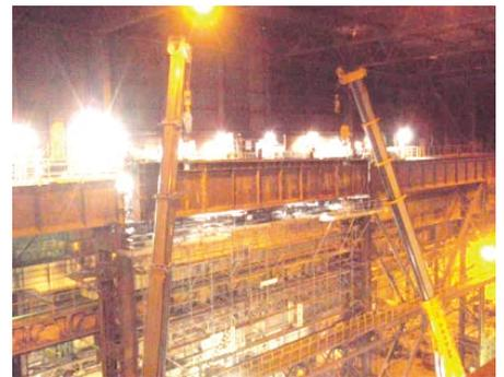
図15: 既設CRG下架
